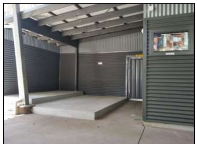
The revised and enlarged viewing area to give Koala Hospital a better view of any procedures being performed.
