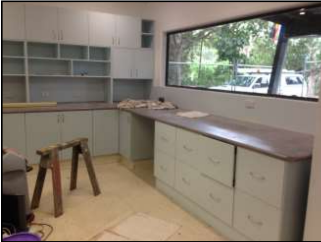
The clinic halfway through the renovation process.
